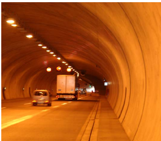
FIGURE 3 Tunnels are important for short connections on Federal Highways (Source: BAST).
