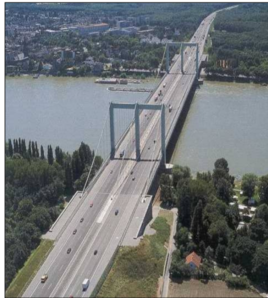
Figure 1 : Bridges are very important infrastructures with a high importance for the road network (Source: BAST)
