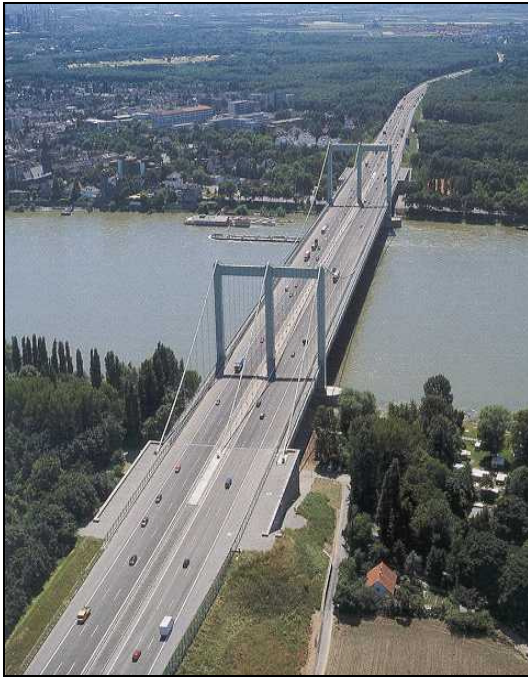
FIGURE 2: Bridges are very important infrastructures with a high importance for the road network (Source: BASt).
